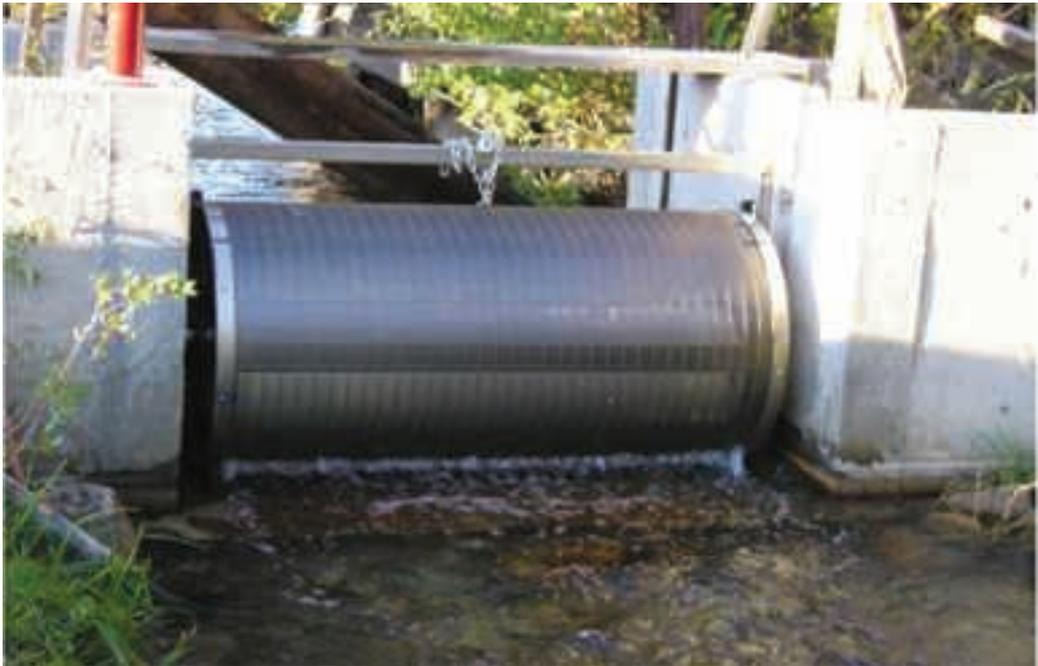
**Fig. 5.3.8. Wedge wire screen cylinder** (photo taken from <http://www.bdiscreens.com/fishdiversion.htm> and used with the agreement of B. Deo-Volente, Inc. 1255 Monmouth Blvd., Galesburg, Illinois 61401).
