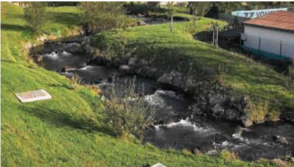
**Fig. 3.8.1.** Example of the bypass channel of the rock-ramp fishway – the complete view (Obermaubach, the Rur River, Germany, photo: D. Bůžek).
