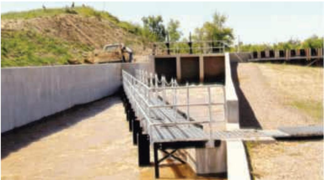
**Fig. 5.3.6. View of the stream of the irrigation channel – inclined position of the barrier – Louvre** (photo taken from [http://www.usbr.gov/pmts/hydraulics\\_lab/pubs/manuals/fishprotection/](http://www.usbr.gov/pmts/hydraulics_lab/pubs/manuals/fishprotection/) used with the agreement of the U.S. Department of the Interior Bureau of Reclamation Denver, Colorado 2006: *Fish Protection at Water Diversions, A Guide for Planning and Designing Fish Exclusion Facilities* 2006, pp. 480).
