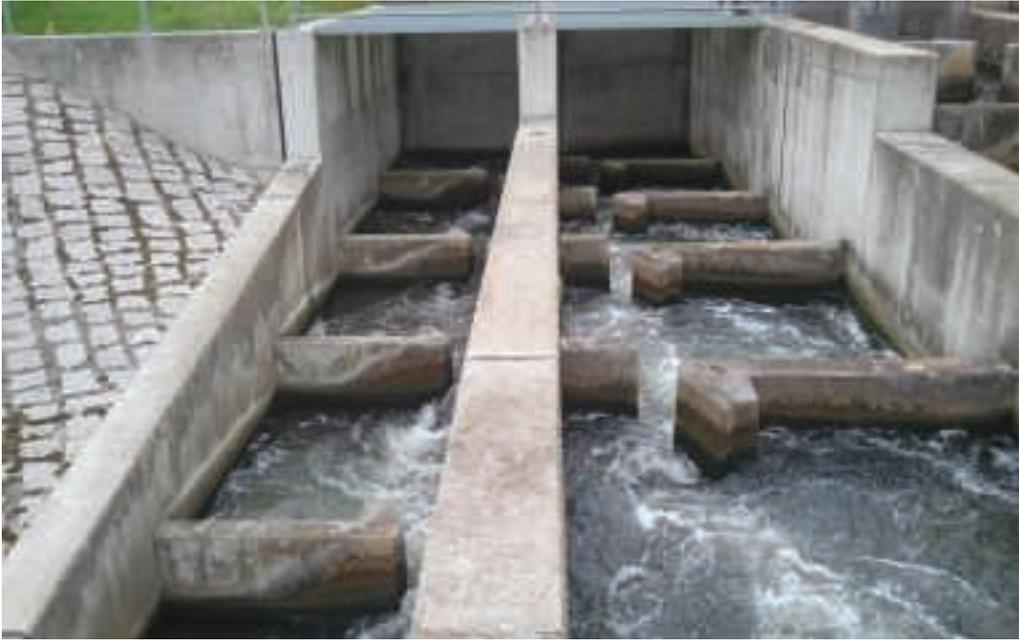
**Fig. 3.8.4.** Details of distribution of main streamlines in the chambers of a vertical slot fishway (Ladenburg, the Neckar River, Germany, photo: M. Drahoňovský).
