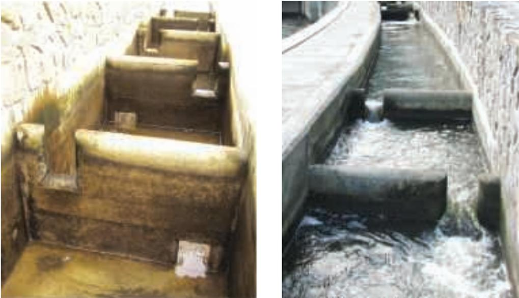
**Fig. 3.8.5.** An example of chamber fishway (Střekov, the Elbe River, Czech Republic, photo: Z. Vančura).
