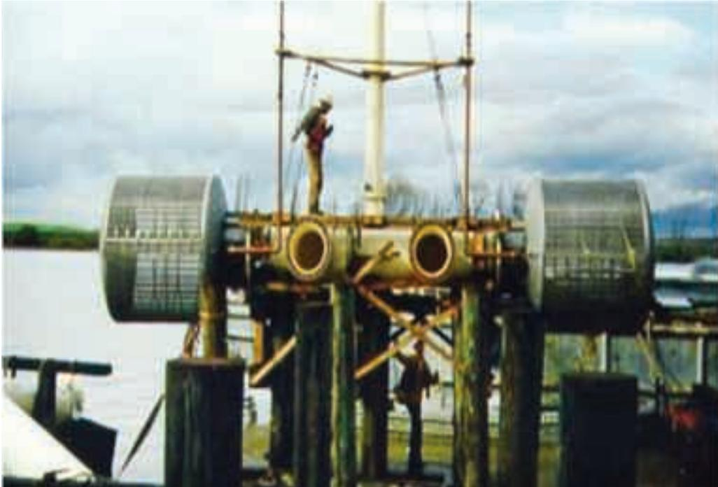
**Fig. 5.3.4.** Cylindrical barrels made of trapezoidal bars installed as a protective filter on piping taking off technological water (photo taken from <http://www.bdiscreens.com/fishdiversion.htm> used with the approval of Industrial Screen Products, Inc., P.O. Box 366, Placerville, CA 95667 USA).
